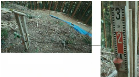
Figure 17 - Monitoring of surface deformation using simple extensometer
