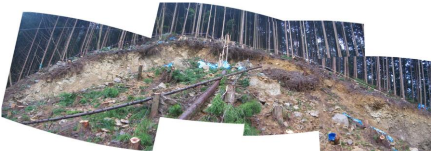
Figure 15 - Typical landslide phenomenon at crest and side, main scarp and lateral scarps are evident
