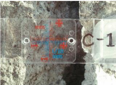
Figure 16 - Monitoring of surface deformation using crack gauge
