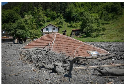
Figure 8- Effects of Flood Floods - Doboj, May 2014 (Photo: Sanja Vrzić)
