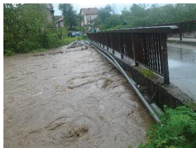
Figure 2- Flash floods in suburban areas of Tuzla during 2010 (Foto: Uljić)
